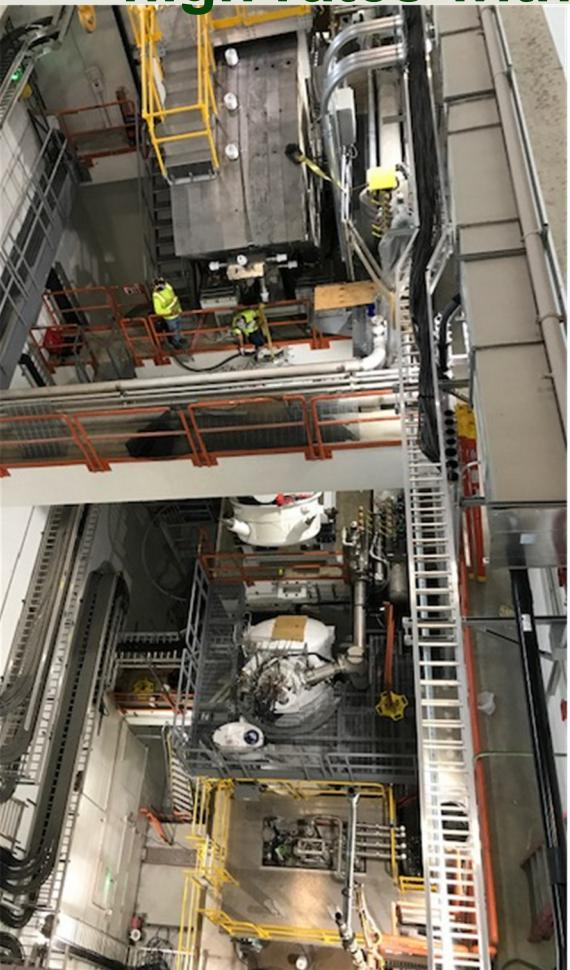
Vertical pre-separator containing a series of SC magnets weighing up to 180 Ton each
