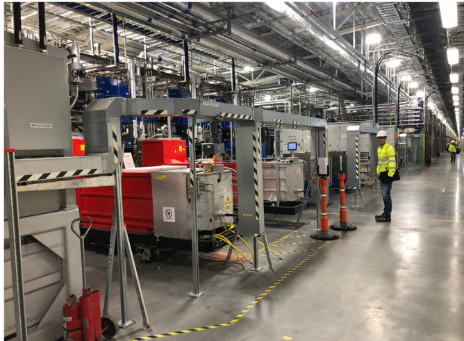
Installation and testing ongoing in superconducting part
